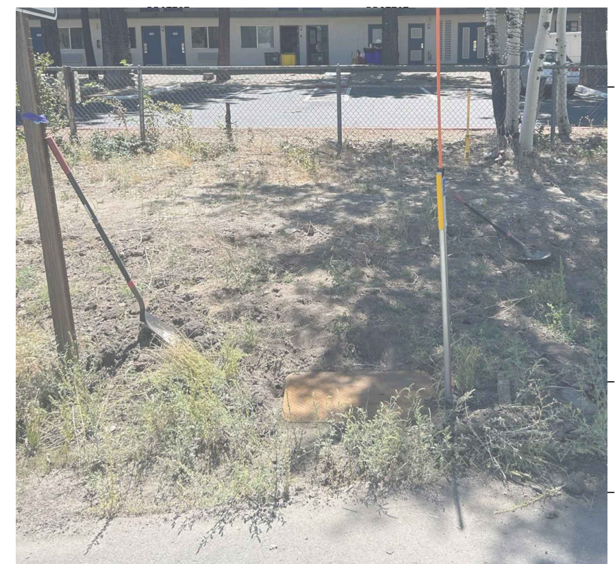
STA 114+36 - 2" SEWAGE COMBINATION VALVE LOCATION PHOTO 2
